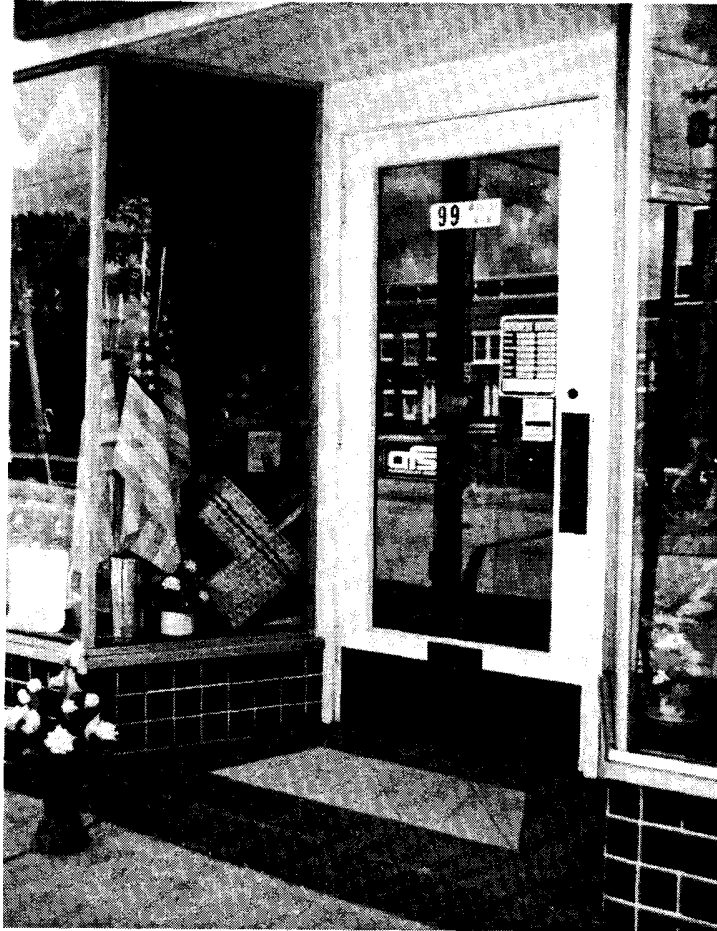
A single door serving a commercial storefront is common practice. This example has no transom but instead has glazing covering nearly the entire door, both to admit light and to permit customers to see into the store.
