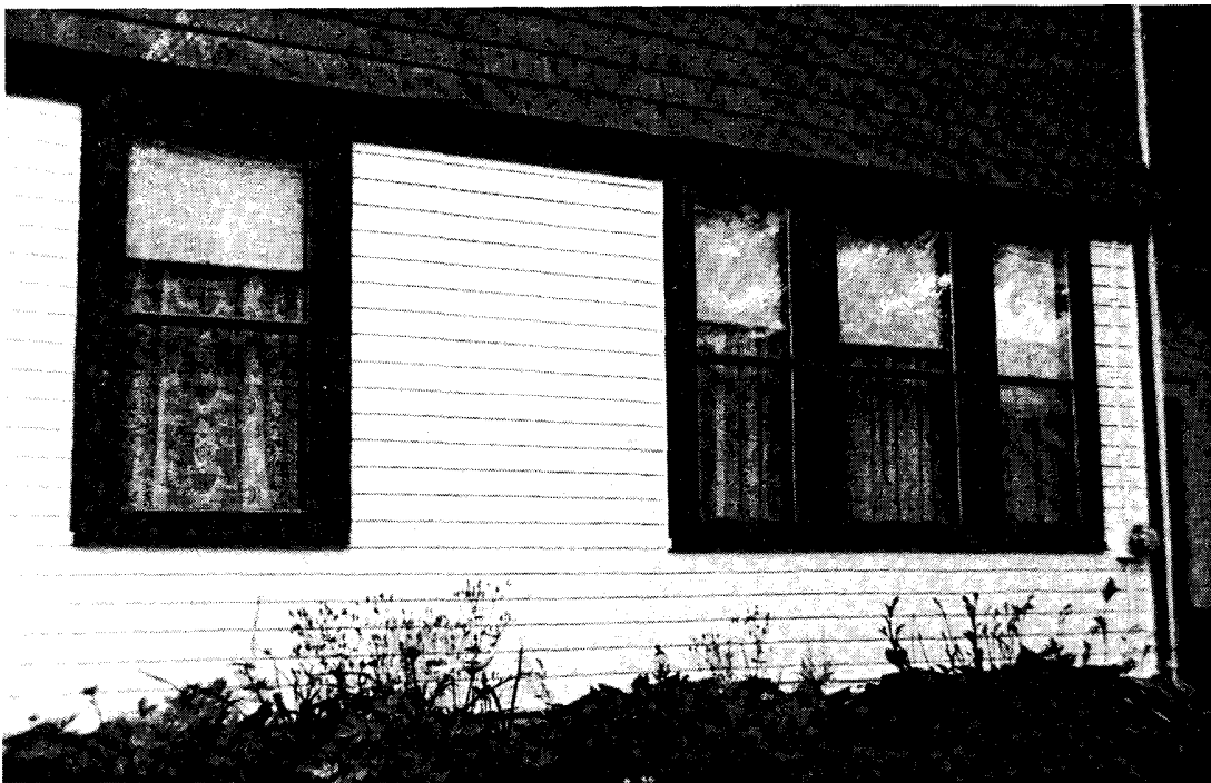
The most common residential window type in Barberton is the double-hung one-over-one sash, which was used throughout the late 19th and early 20th centuries. In this house, both single and clustered windows provide variety in the architectural design.
