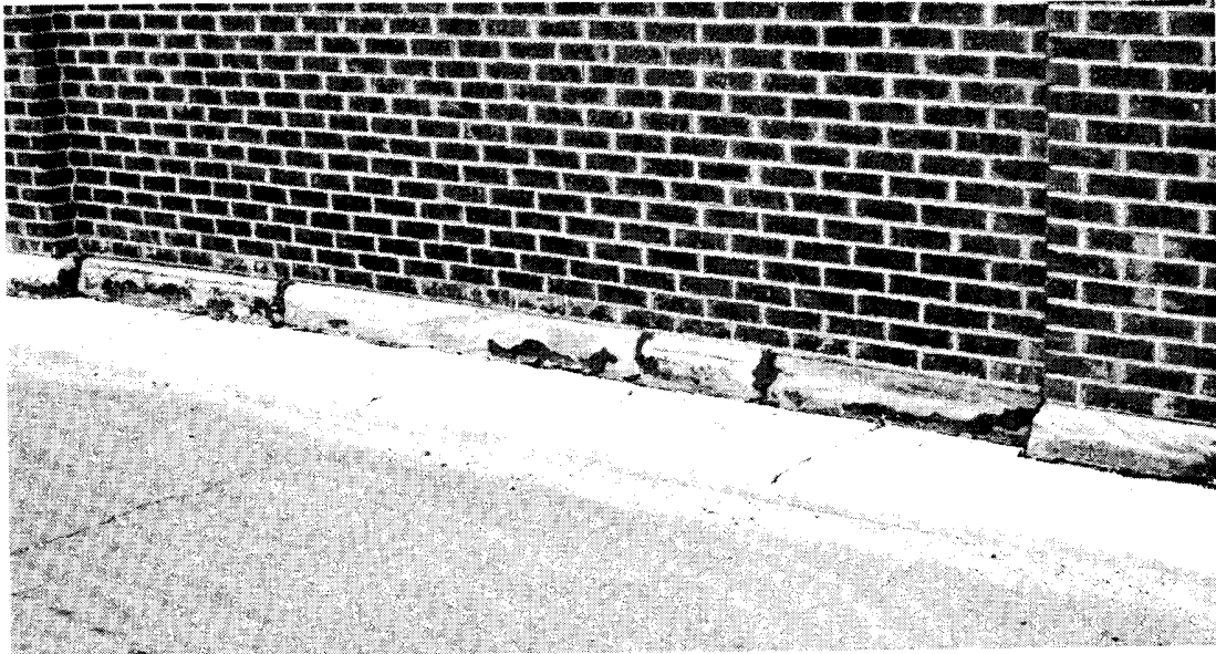
Most building foundations are either invisible or can barely be seen, as in this downtown Barberton example. The roughly-finished stone is a typical foundation material.
