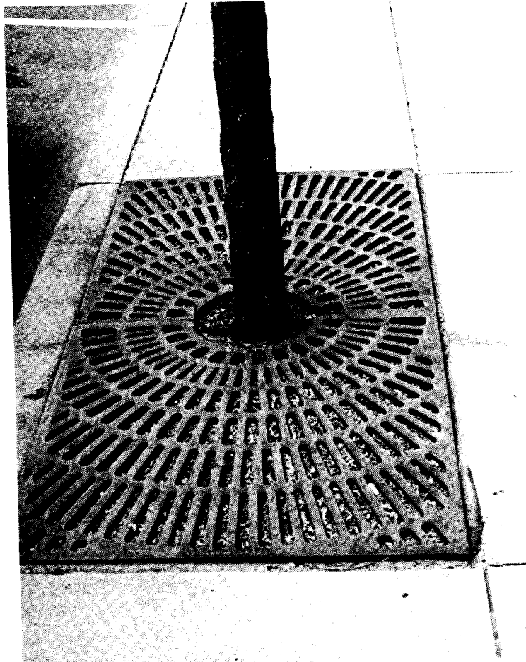
Cast iron tree grates help provide a smooth walking surface but also admit rainwater for the tree. The trunk hole can be enlarged as the tree grows.
