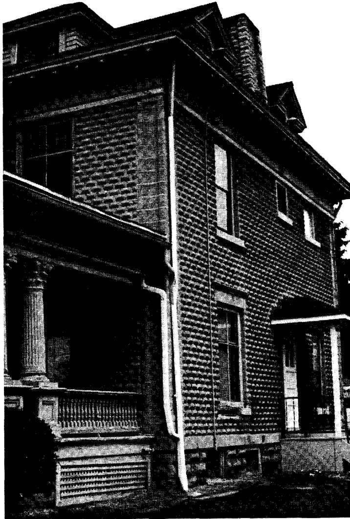
This Barberton house is built of a distinctive rock-faced concrete block that gives it a solid feel and a highly textured surface. Note the different block used to define the corners.
